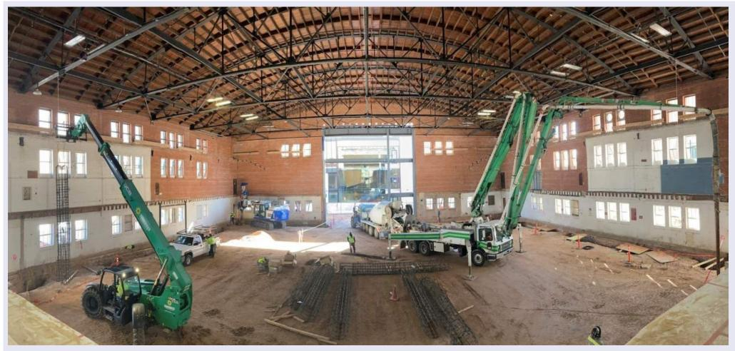
View of progress in January from inside the main entrance looking south. The large equipment installing rebar columns provides some perspective of the spacious interior. The windows of the completed Bartlett Academic Success Center are visible beyond.
