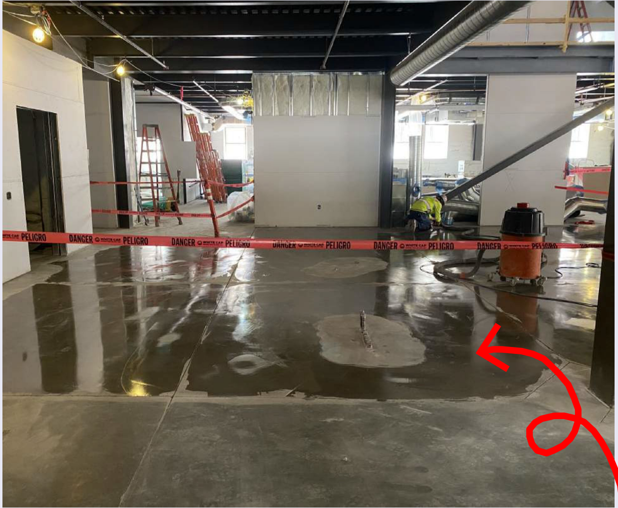
On the left, mechanical ductwork is being installed above the existing historic gym floor and bleachers. On the right, the level one concrete slab on grade is being polished. On top of this polished floor will be the reception desk for a wellness lounge and studio.
