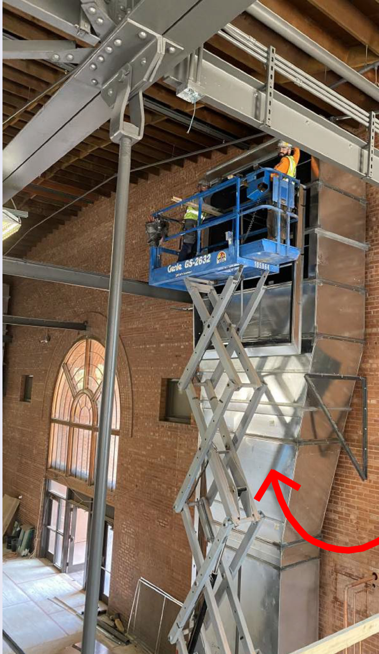
On the left, mechanical ductwork is being installed above the existing historic gym floor and bleachers. On the right, the level one concrete slab on grade is being polished. On top of this polished floor will be the reception desk for a wellness lounge and studio.
