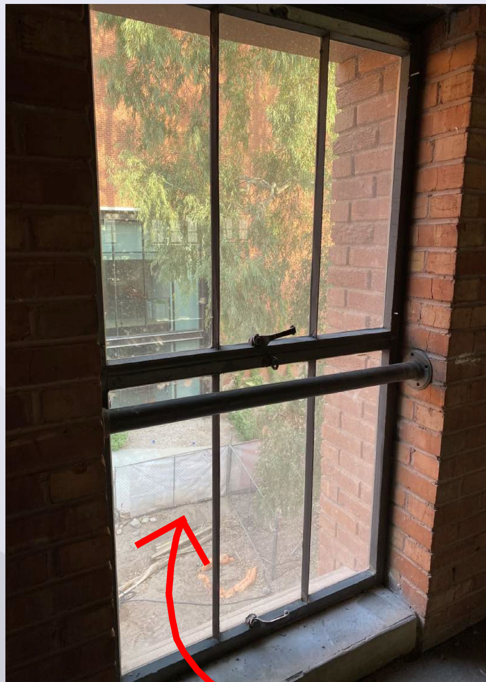
On the left, one of 184 windows has received new glazing putty and glass. The historic steel frames will remain. On the right, footings are being prepped for steel canopies that will span between the Main Library and the Bear Down Gym.
