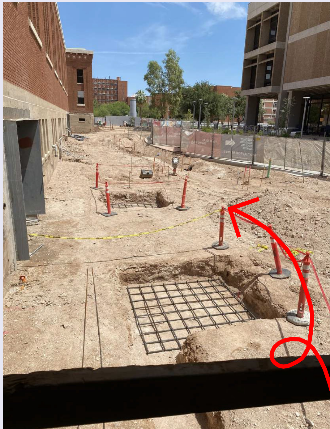
On the left, one of 184 windows has received new glazing putty and glass. The historic steel frames will remain. On the right, footings are being prepped for steel canopies that will span between the Main Library and the Bear Down Gym.
