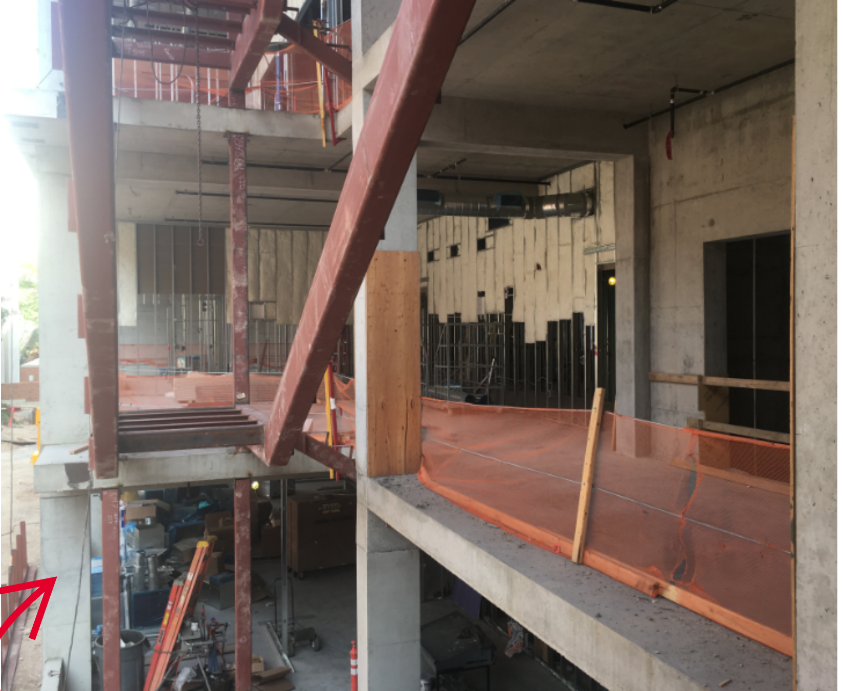
THE BARTLETT ACADEMIC SUCCESS CENTER MAIN STAIR STEEL IS BEING INSTALLED!
