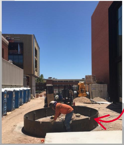
VIEW OF HARDSCAPE WORK TO THE NORTH OF MAIN LIBRARY POD 'A'. BRICK HAS BEEN REMOVED FOR NEW CONCRETE BANDS TO BE INSTALLED
