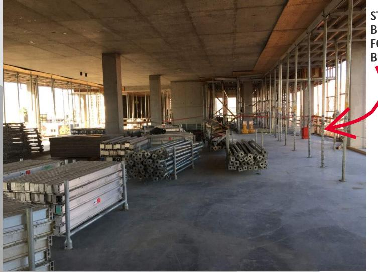
STUDENT SUCCESS BUILDING LEVEL 4 FORMWORK IS BEING STRIPPED!
