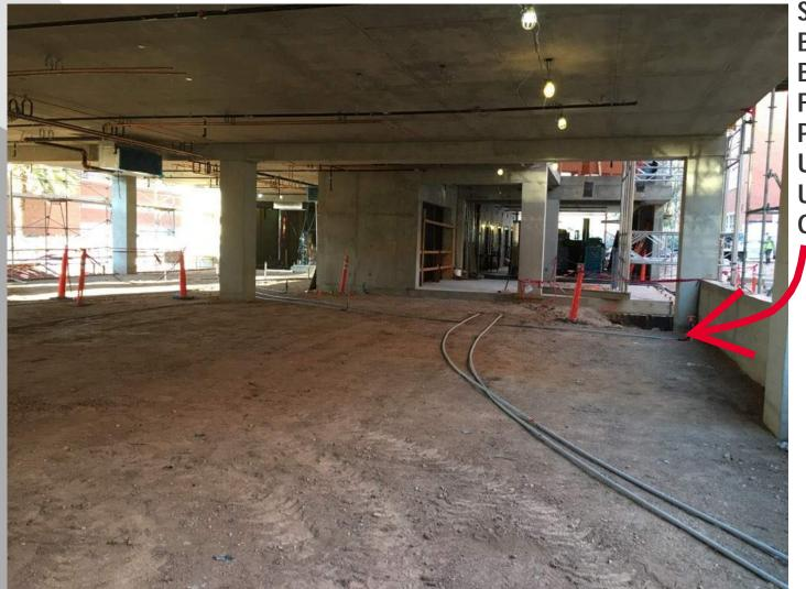
STUDENT SUCCESS BUILDING LEVEL 1 IS BEING PREPARED FOR SLAB ON GRADE PLACEMENT WITH UNDERGROUND
