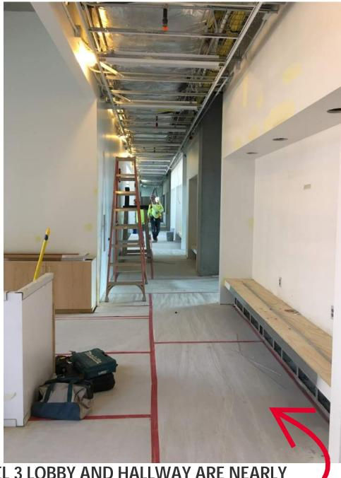
BARTLETT ACADEMIC SUCCESS CENTER LEVEL 3 LOBBY AND HALLWAY ARE NEARLY COMPLETE AND READY FOR FLOOR PROTECTION TO BE REMOVED AND CONCRETE TO BE POLISHED! WOOD SLATTING IS BEING FITTED AT ELEVATOR FRONTS - BEFORE BEING REMOVED AND ETCHED WITH THE FLOOR DESIGNATION!
